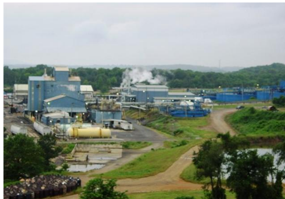
U.S. Vanadium's Processing Facility in Hot Springs, Arkansas USA
