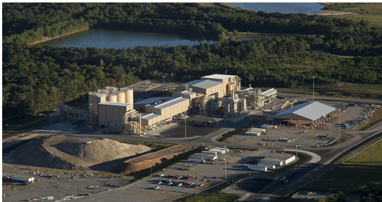
Benton, Arkansas processing facility
